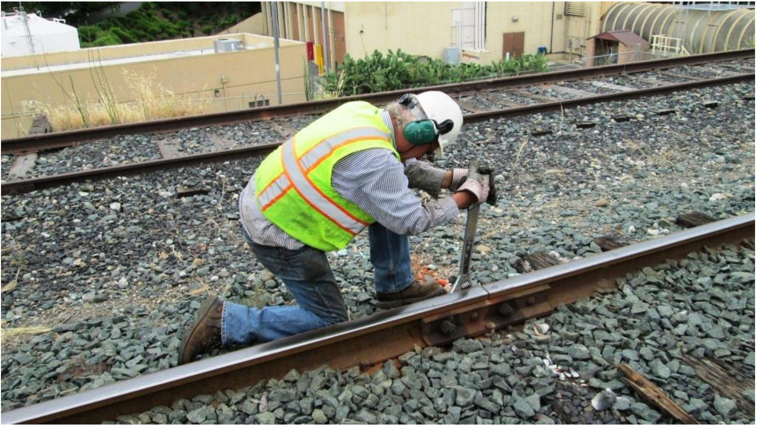
Steve tightens down a new bolt in a track joint
