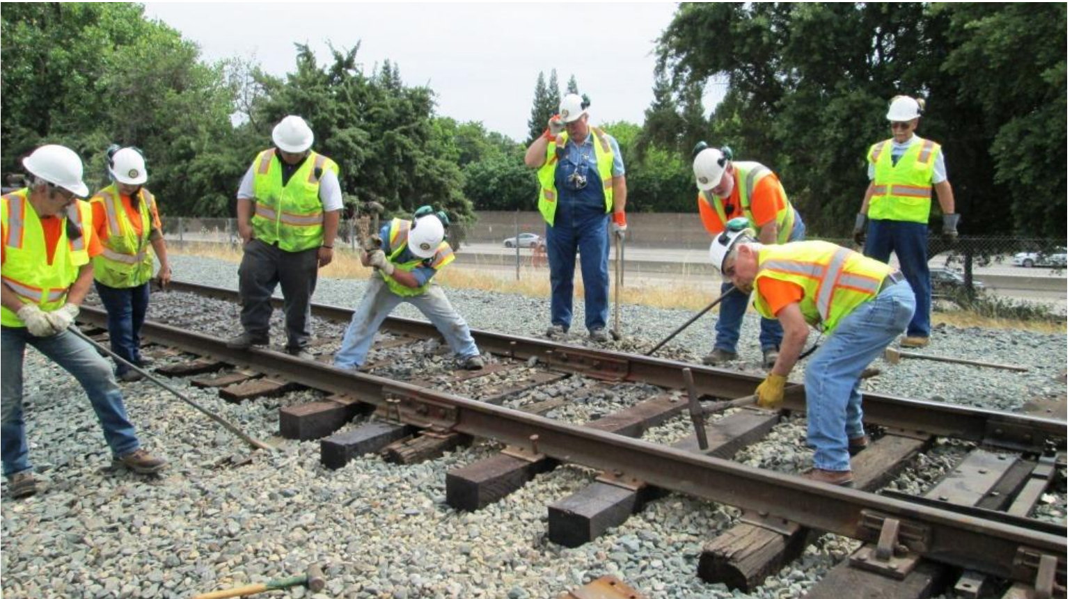
Frank and Ed K. nip the ties as Joe and Mike W. drive spikes
