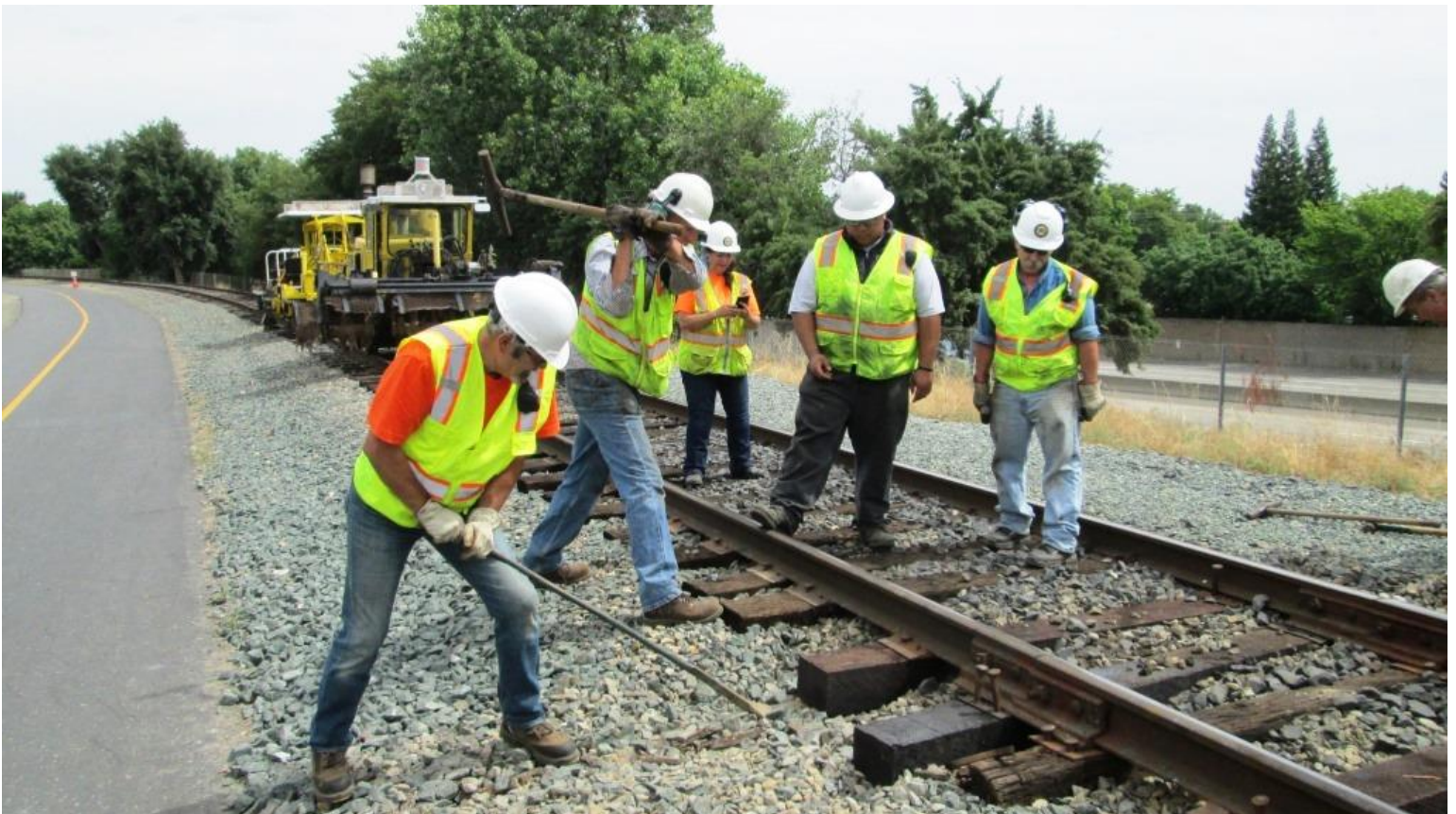
We've come full windmill with Steve driving more spikes while Ed K. nips the tie
