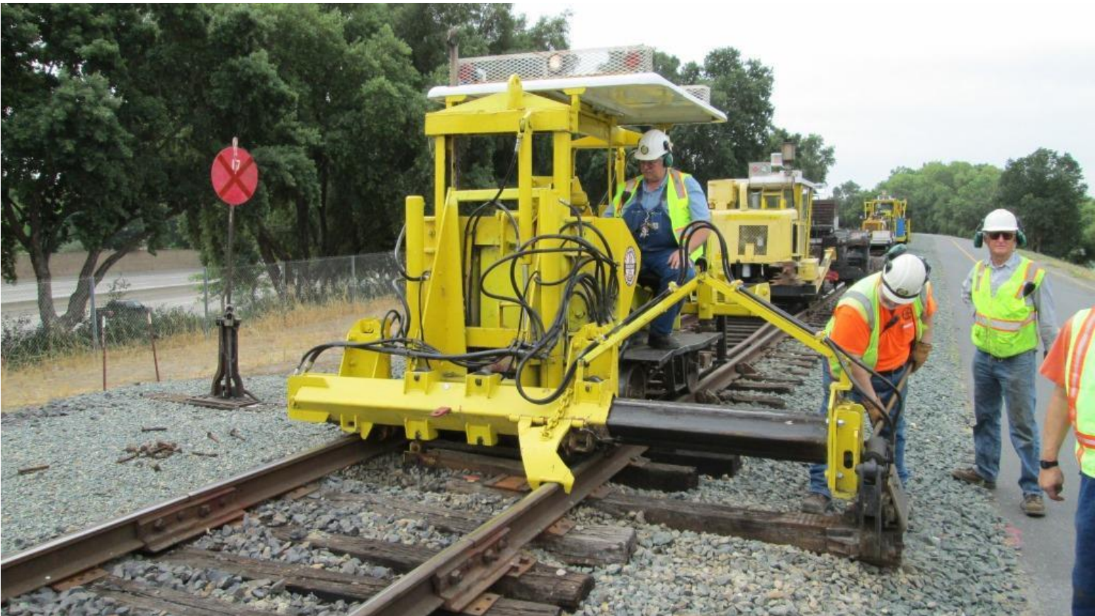
Frank keeps rock from mounding at the end of the tie that Chris is pulling with the Jackson 125
