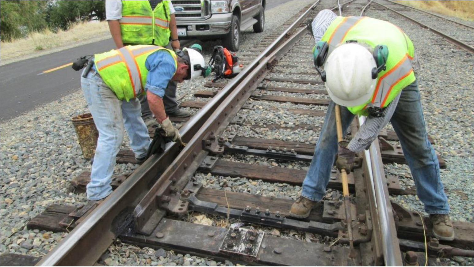
Joe applies grease to the plates while Steve scrapes off more gunk
