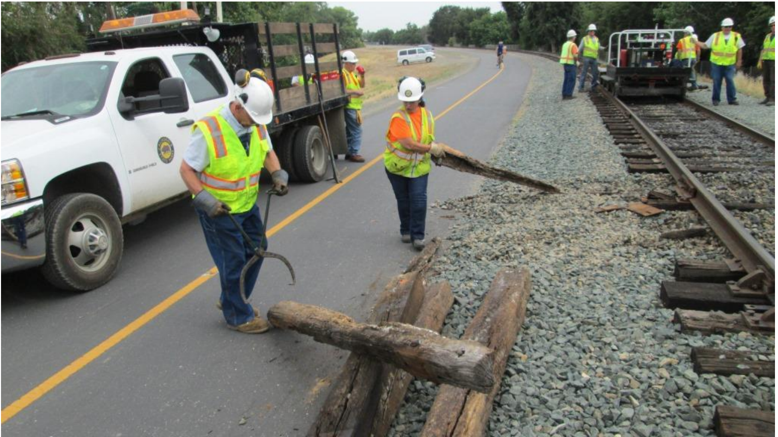
Clem and Pam remove the remnants of the pulled ties. As you can see, they kind of disintegrated as they were pulled
