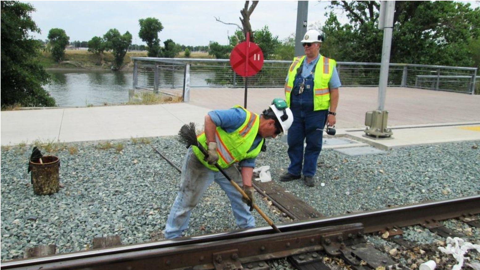
Chris, with oil-can in hand, oils the switch-machine while Joe scrapes gunk off the switch-plates
