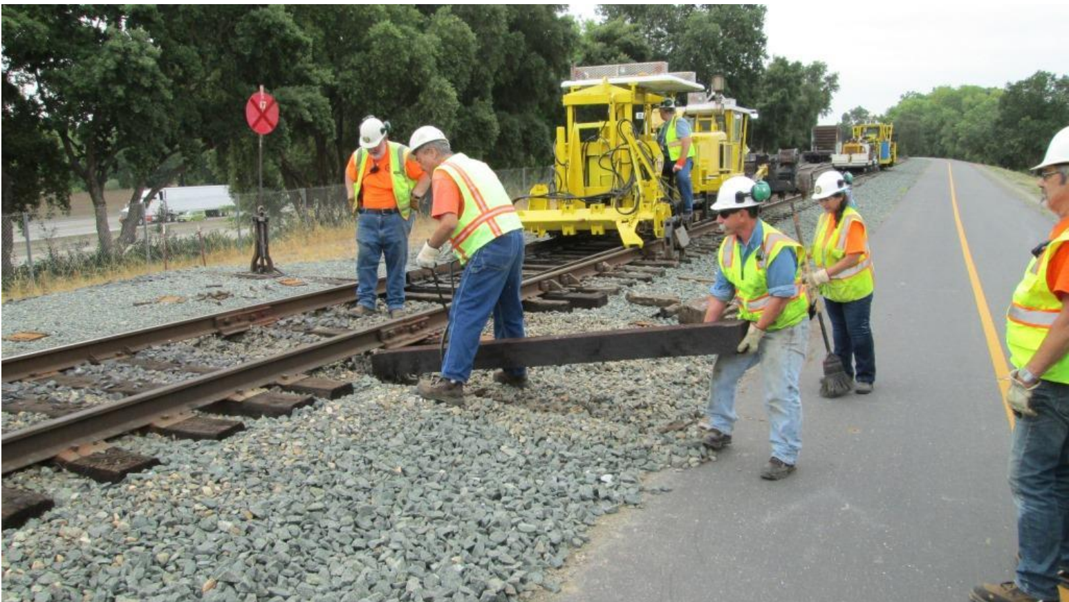
John and Joe set a new tie for insertion
