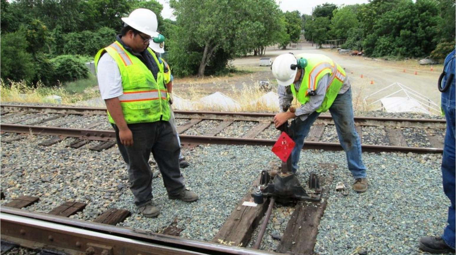
With the switch serviced, Steve tests the operation of the ground-throw switch #13
