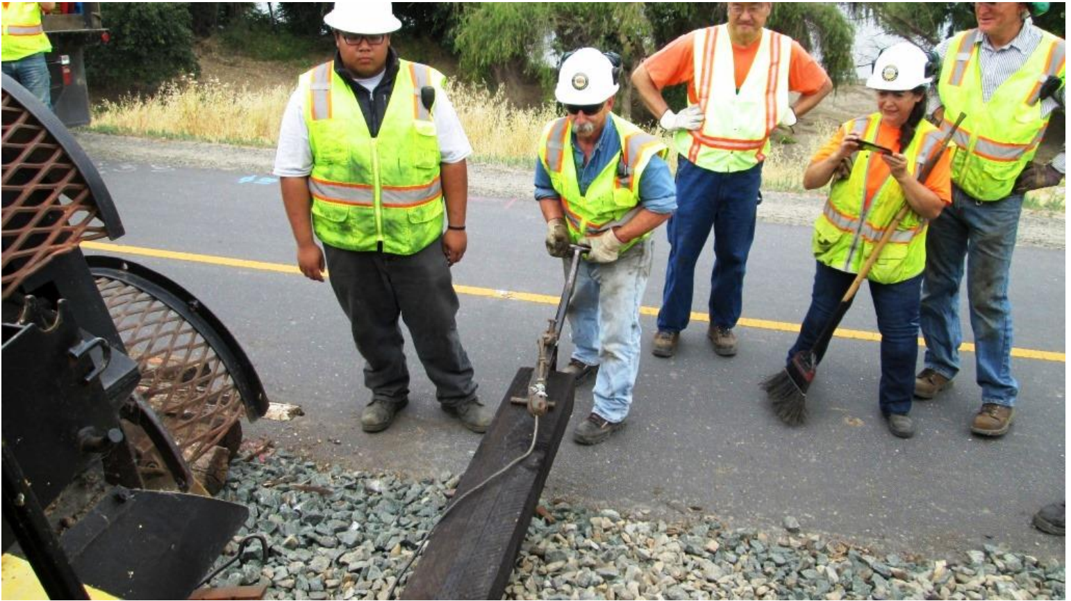
The view from inside the scarifier as Joe guides the insertion of a tie
